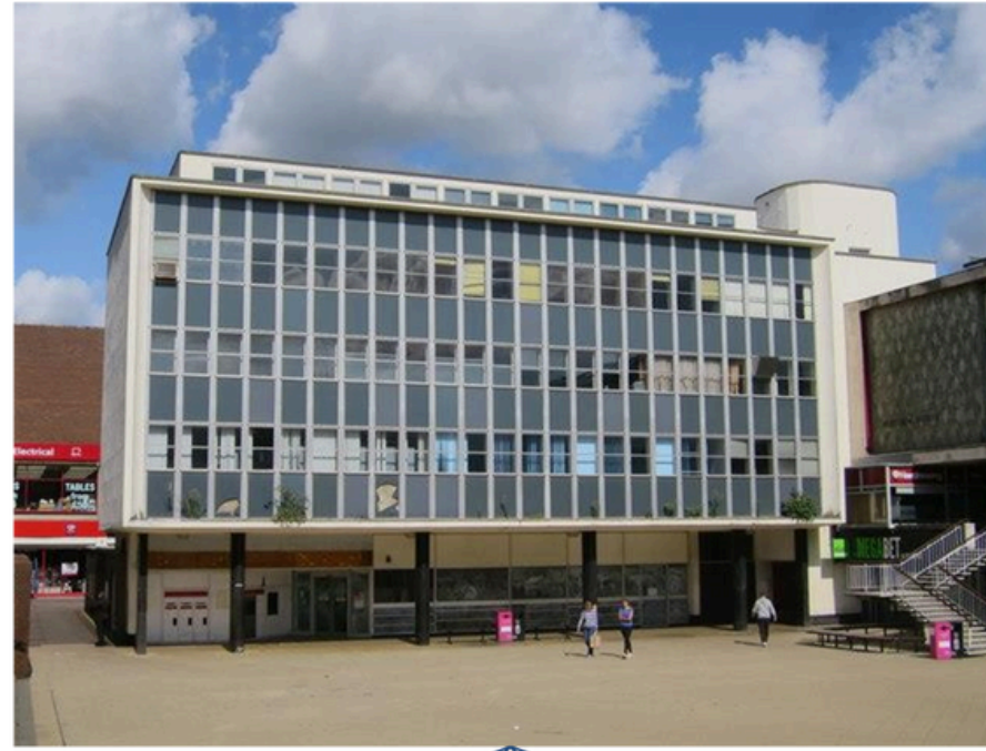
Headquarter Office/ Corporate Office
